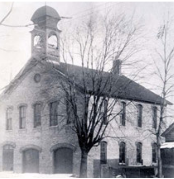
Engine House, c. 1915
